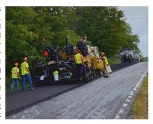
At the end of the CIPR process the roadway is rolled and is then ready to be topped with a wearing course overlay of a hot mix, warm-mix, cold mix or chip seal product. Unique to our CIPR process, the Roadtec RX900E is the same length as a conventional milling machine with an attached loading conveyor enabling us to work in areas not compatible for most other equipment.
